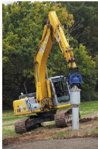
▲ Installing a screw foundation for a dual-axis tracking system (Deger-Traker) at Am Peterswald PV park in Germany: Bftec GmbH pre-drills the ground at the site and then the foundation is installed. The foundation's unusual form, which consists of a smooth side wall with a coil at the bottom (if necessary, two coils), guarantees a firm grip. The foundation can rotate in the ground without displacing or loosening the surrounding earth.
