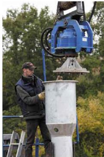
▲ Installing a screw foundation for a dual-axis tracking system (Deger-Traker) at Am Peterswald PV park in Germany: Bftec GmbH pre-drills the ground at the site and then the foundation is installed. The foundation's unusual form, which consists of a smooth side wall with a coil at the bottom (if necessary, two coils), guarantees a firm grip. The foundation can rotate in the ground without displacing or loosening the surrounding earth.
